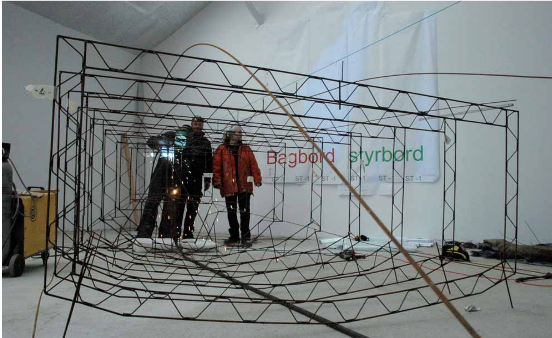
Full scale production of the armature.
