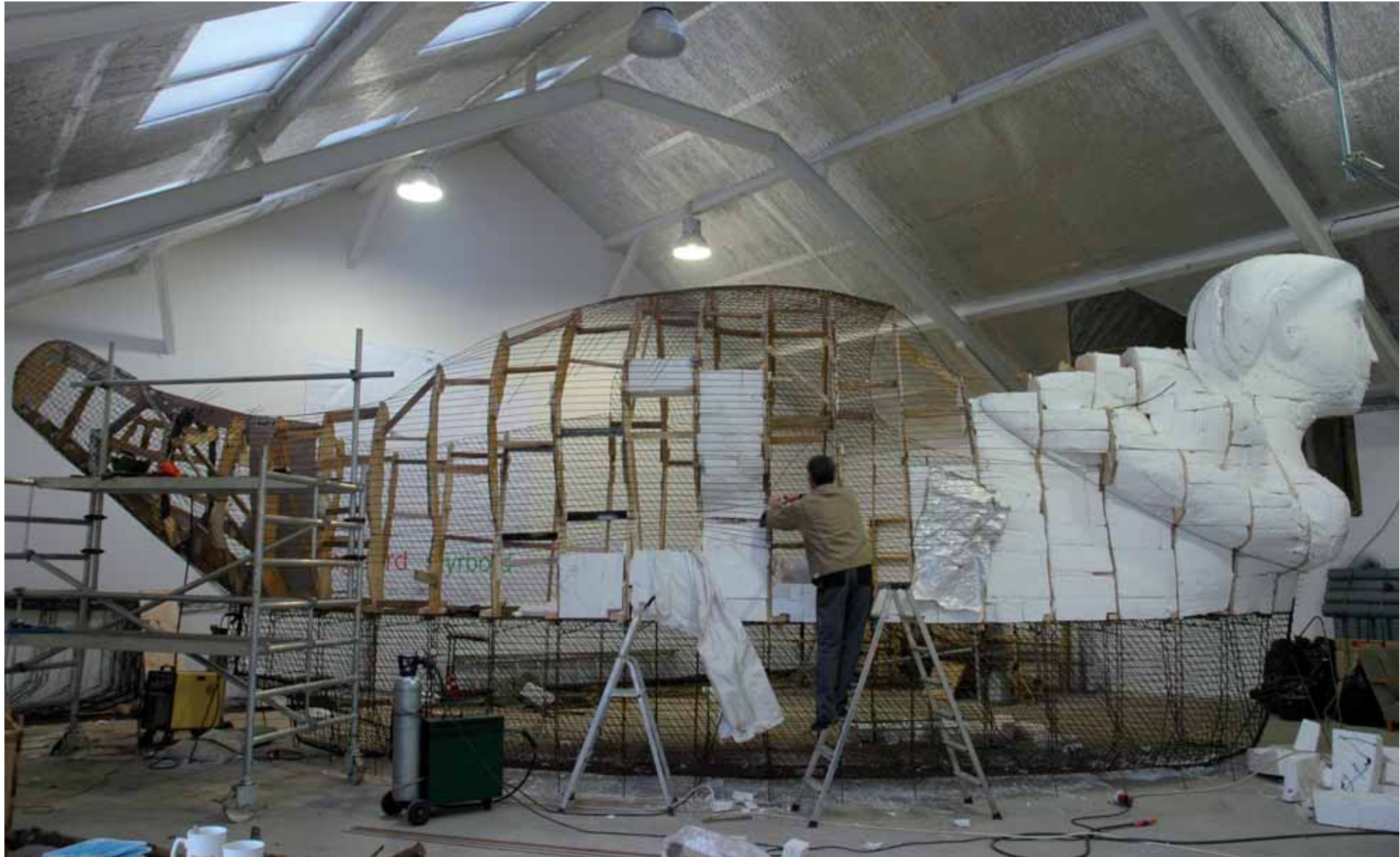
The framework in wood, with a polystyrene filling to shape the body, which will be removed after the rest of the body has been welded with transverse and diagonal steel reinforcement
