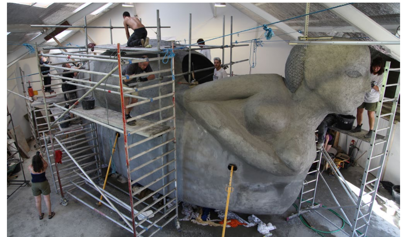
BUILDING PROCESS IN MYGDAL SHIPYARD
